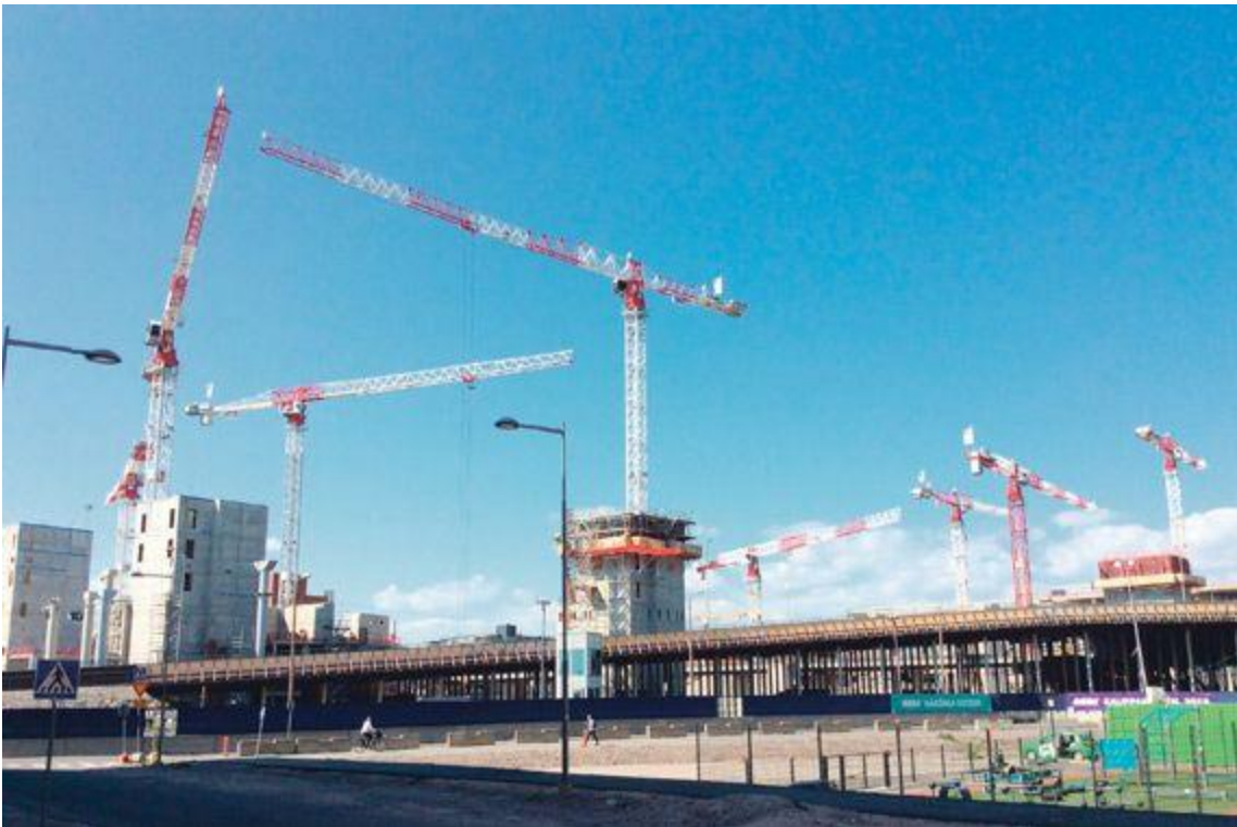
The new Kalasatama neighborhood is currently under construction.
